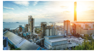
INDUSTRIAL AND STATIONARY EQUIPMENT
